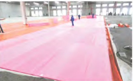
Cold Storage Floor
